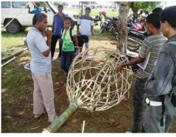
Bracing slats at 45 degrees are then tied in with similar steel wire.
