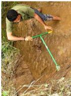
Normally, the gabions will stay much longer in place if they are anchored with retainers made of 6 mm steel reinforcement bars. For this purpose 10-12 cm wide holes are horizontally bored 1 meter into the riverbank or the hill slope with a hand auger. This tool can easily be manufactured in a local metal workshop from a 10 cm wide regular steel tube.
