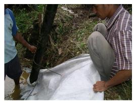
Protection by gabion stone cages can be further improved with geotextile tissue which lets water flow through but retains the soil particles. This will no doubt help to avoid soil being eroded behind the stone filled gabions.
